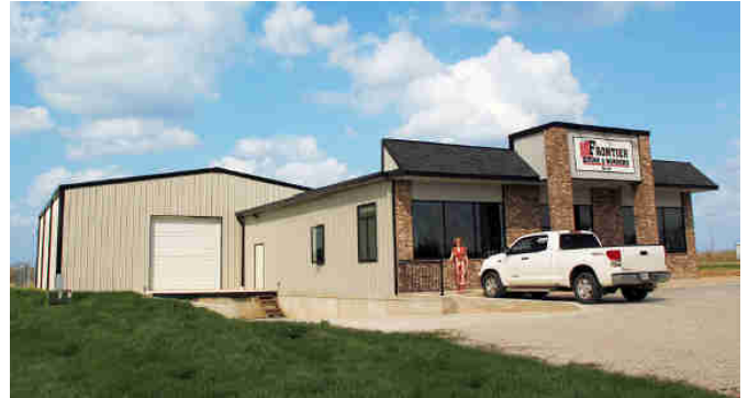
Frontier Siding Company in Stillwater, Oklahoma. Both buildings are bolt up, light Stone walls with Burnish Slate trim.
